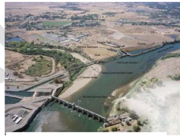
Image 2 – TCCA Pumping Plant
