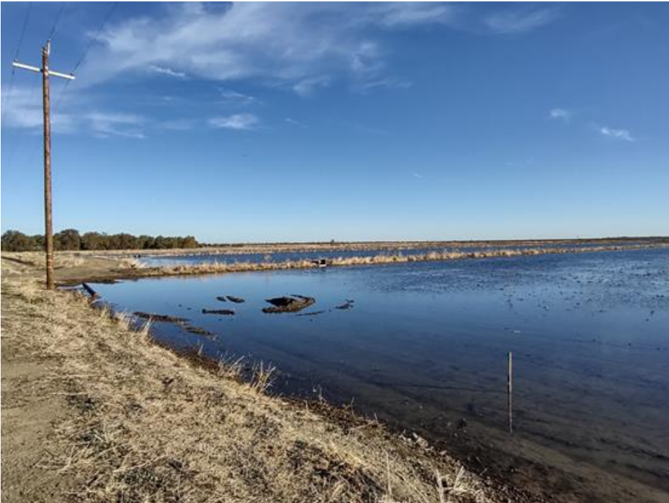
Field 4 flooded (from November 3 rd )
